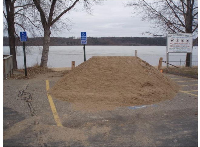
Sand placed at river embankment for pending sandbagging operations
