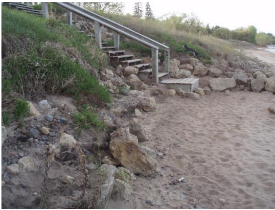
Post flood erosion damage to area around north beach stairway
