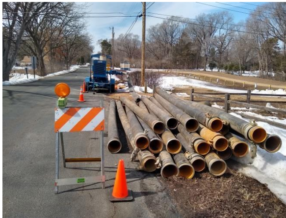
Hard casing discharge hose is stationed and ready for deployment when needed
