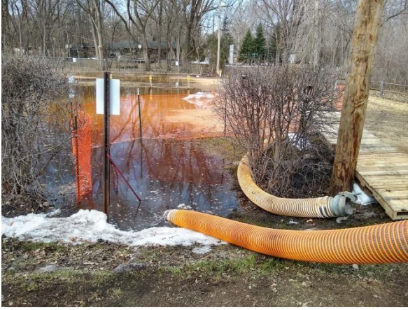
Intake hose is station and set-up at beach parking lot culvert
