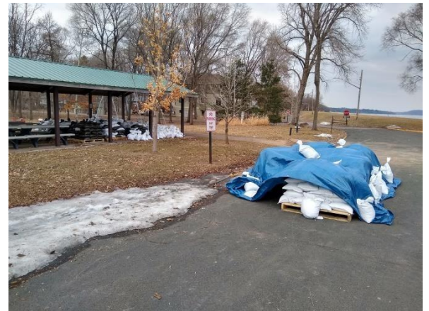
Sandbags are positioned under pavilion and covered so they don't absorb rain
