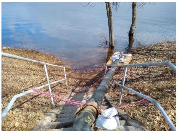
Last section of hard casing discharge hose is secured to staircase with 90 degree elbow pointed up attached at end
