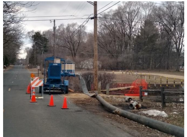
Collapsible hose is connected to discharge port and then connected to hard casing discharge hose
