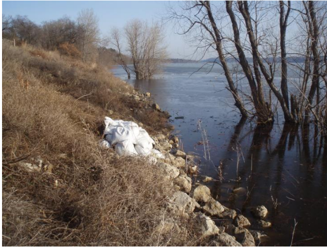
Sandbagging 17 th St. flapgate as water approaches base of drain culvert
