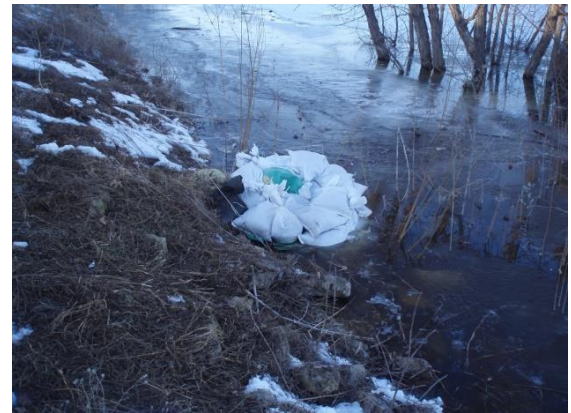
Sandbags hold down 17 th St. flapgate
