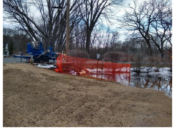
Fencing is placed around suction area to hold back debris from entering intake
