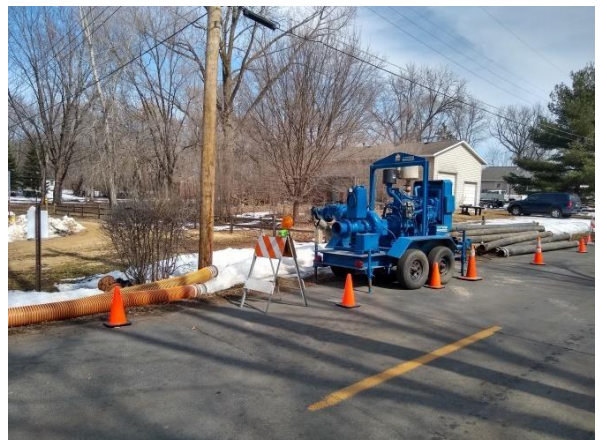
8" pump is delivered with more than 400 feet of intake and discharge hose
